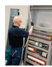
Designed and manufactured in-house, our motor control centres are constructed to the client's specification or, if preferred, we will select the most appropriate equipment to meet the projects exact requirements. From form 2 to form 4, types 1-7, local or remote, manual or automatic control, all our control systems are rigorously tested to ensure correct performance and compliance.
